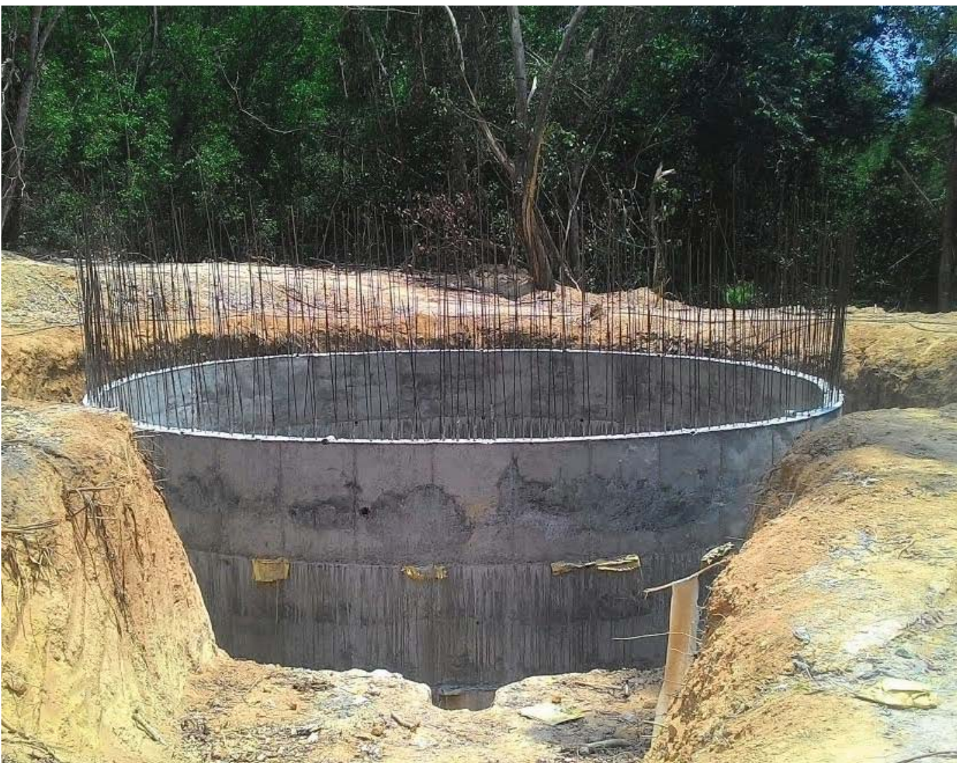
The well which is being constructed near the Haimavathy Pond
